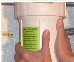
Replace each filter cartridge into sump. Hand tighten sump into housing.
