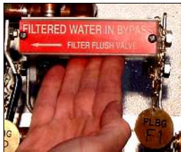
Move F1 handle up to "Filtered Water in Bypass" position.
