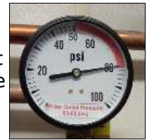
Outlet Gauge Peaks Between 50-80 psi
