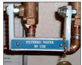
Close valves F4 and F2. Return valve F1 to "Filtered Water in Use".
