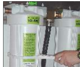
Remove each sump using sump wrench. Rinse each sump with mild soap solution.
